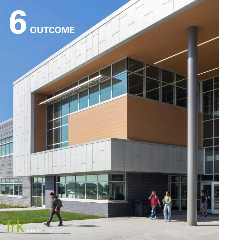
The design team collaborated closely with the owner and local energy company, conducting energy modeling and lifecycle analysis for proposed building systems. Northwest High School achieved a verified 35% reduction in Energy Use Intensity (EUI) compared to code-level buildings, resulting in approximately \$140,000 in annual operational savings. Additionally, the building received a \$231,000 rebate through energy company rebate systems to offset initial cost increases.
