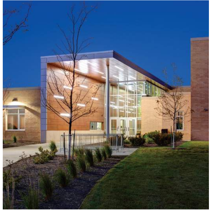
The exterior façade of the building is comprised of masonry, prefinished metal, and phenolic composite wall panels, providing both durability and aesthetic interest to this neighborhood school.
